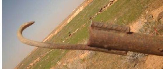
The damaged Heavy rake
